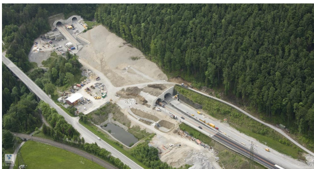
Aerial view, Leipzig Tunnel.
