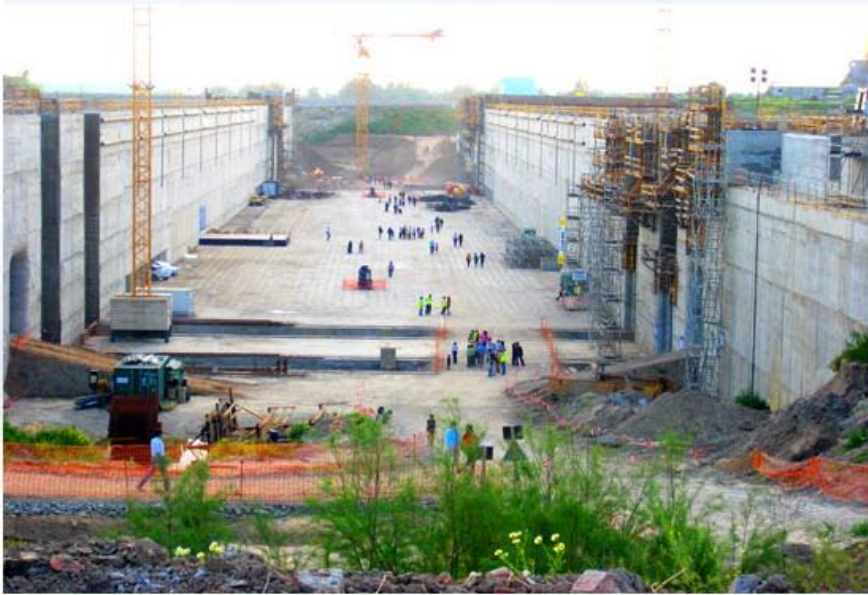
Navigation channel. New lock at Seville Harbour.
