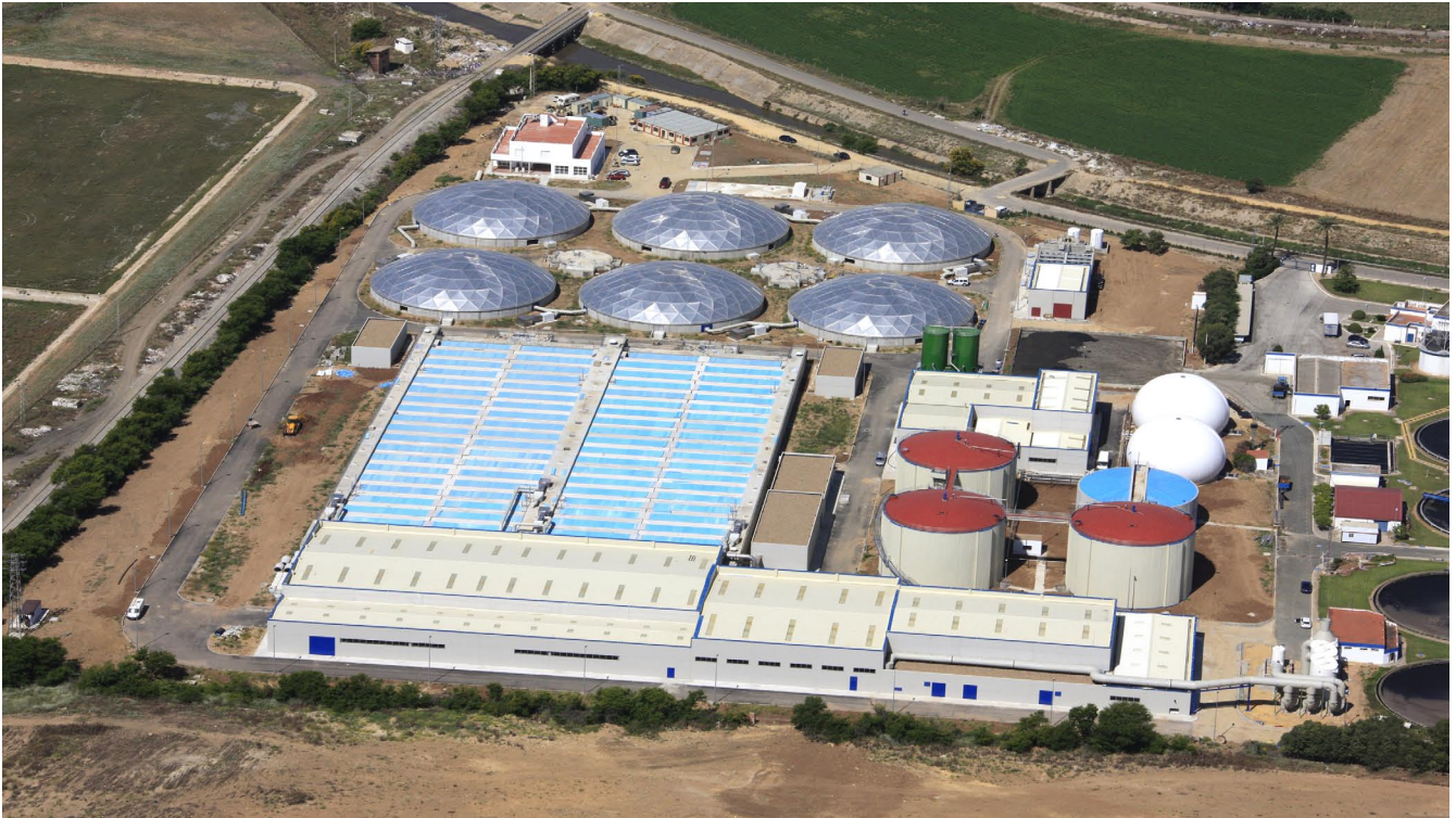
New Ranilla wastewater treatment plant. Seville.
